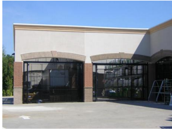
Figure 9-B: The above image illustrates a wall and fence that is an extension of the principal building that is designed to screen outdoor storage areas.
