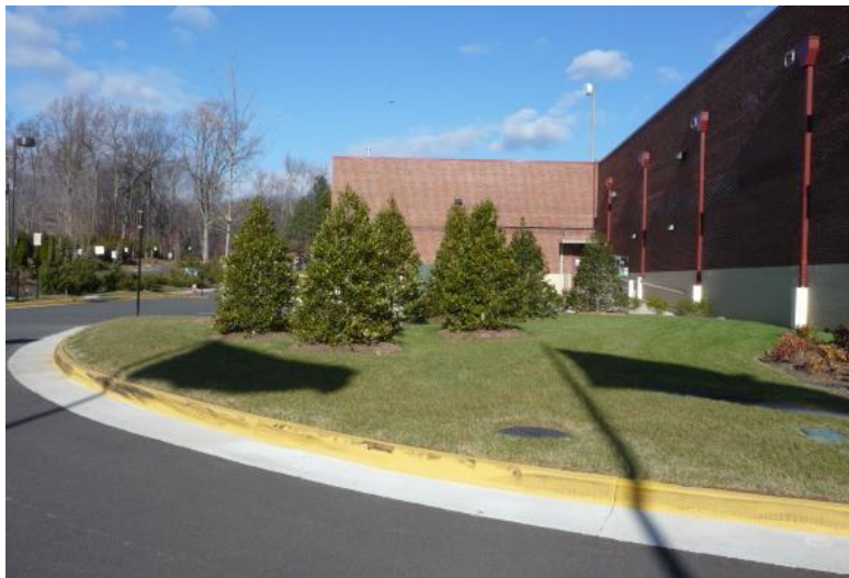
Figure 9-A: The above image illustrates a vegetative screen that hides HVAC equipment and a dumpster.
