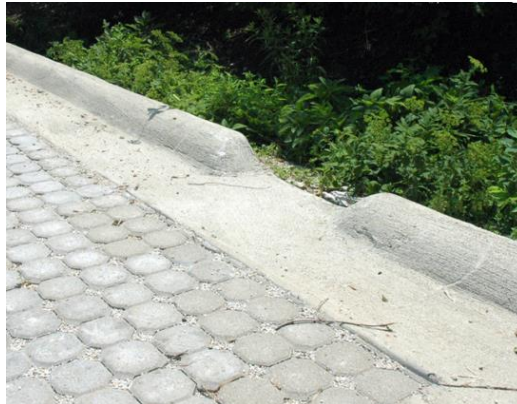
Figure 10-A: Cuts in the continuous curb allow for stormwater to be directed into landscaped areas.
