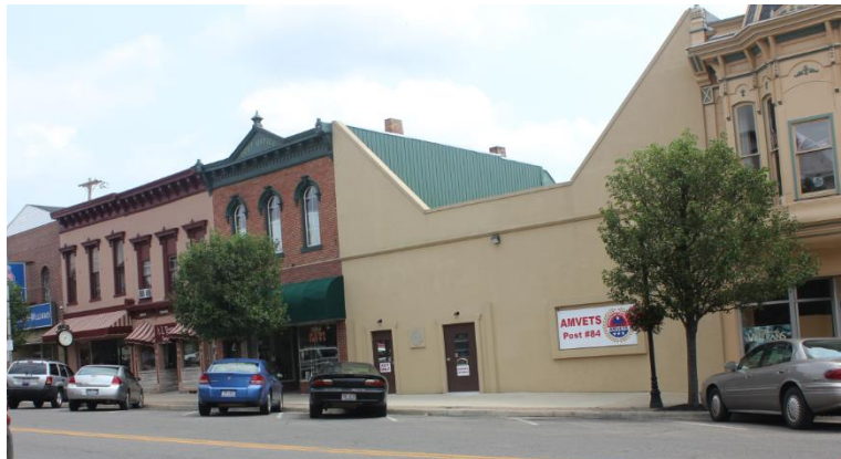
Figure 8-E: This image illustrates an infill building that would not comply with these standards of new construction in terms of height, roof styles, window and door patterns, siding, ornamentation, and signage.
