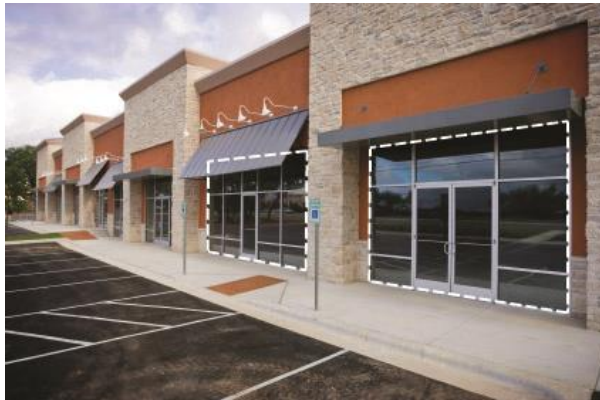
Figure 11-I: The window area is illustrated within the dashed line area for the two storefronts in the above image.
